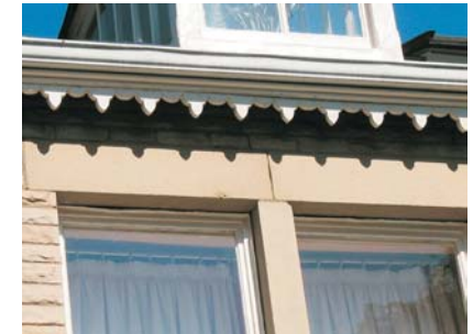
(l) Stone sills and lintels.
